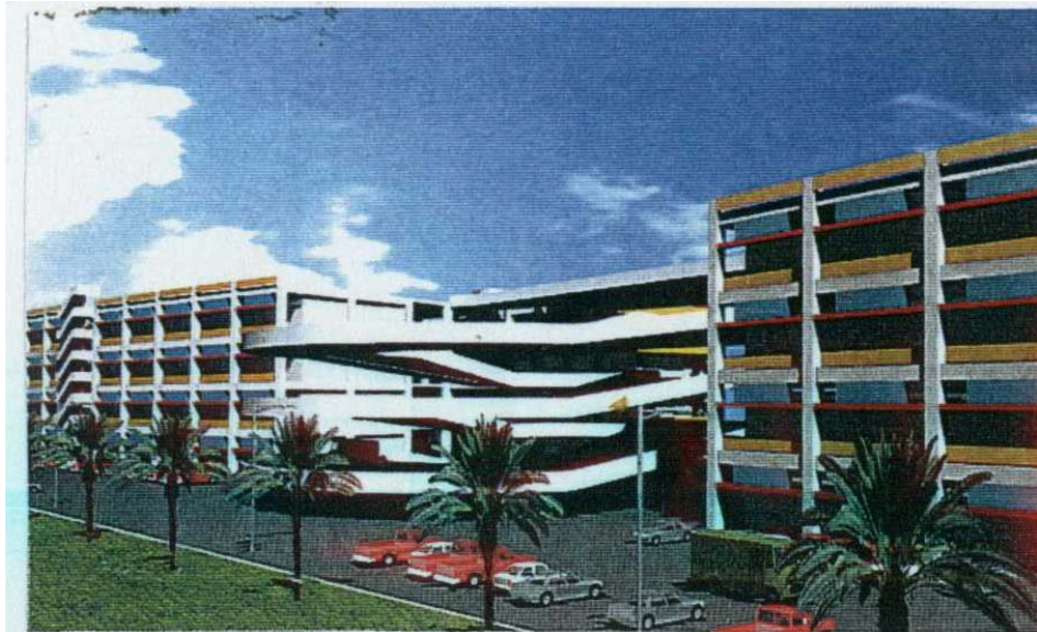
Drive-up factories at Woodlands Link Fast track construction with precast columns/beams double-T
