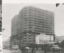
Tsong Wei Building, Taipei 榮偉大廈
