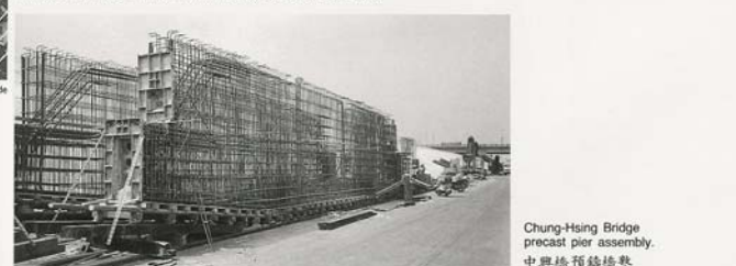
Chung-Hsing Bridge precast pier assembly 中興橋預鑄橋墩
