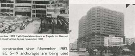
Tsong Wei Building, Taipei 崇偉大廈
