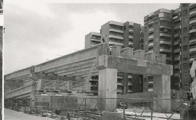
Chung-Yang Bridge during erection 重陽大橋台北引道部份
